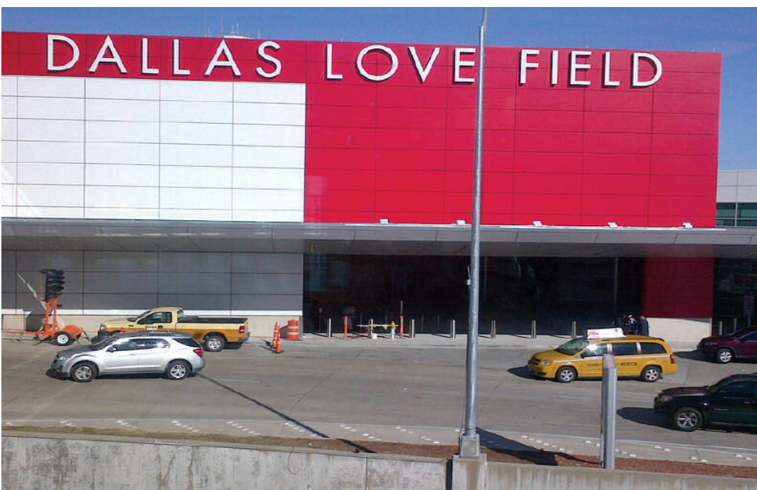
Entrance into Terminal 2 via curbside check-in.
