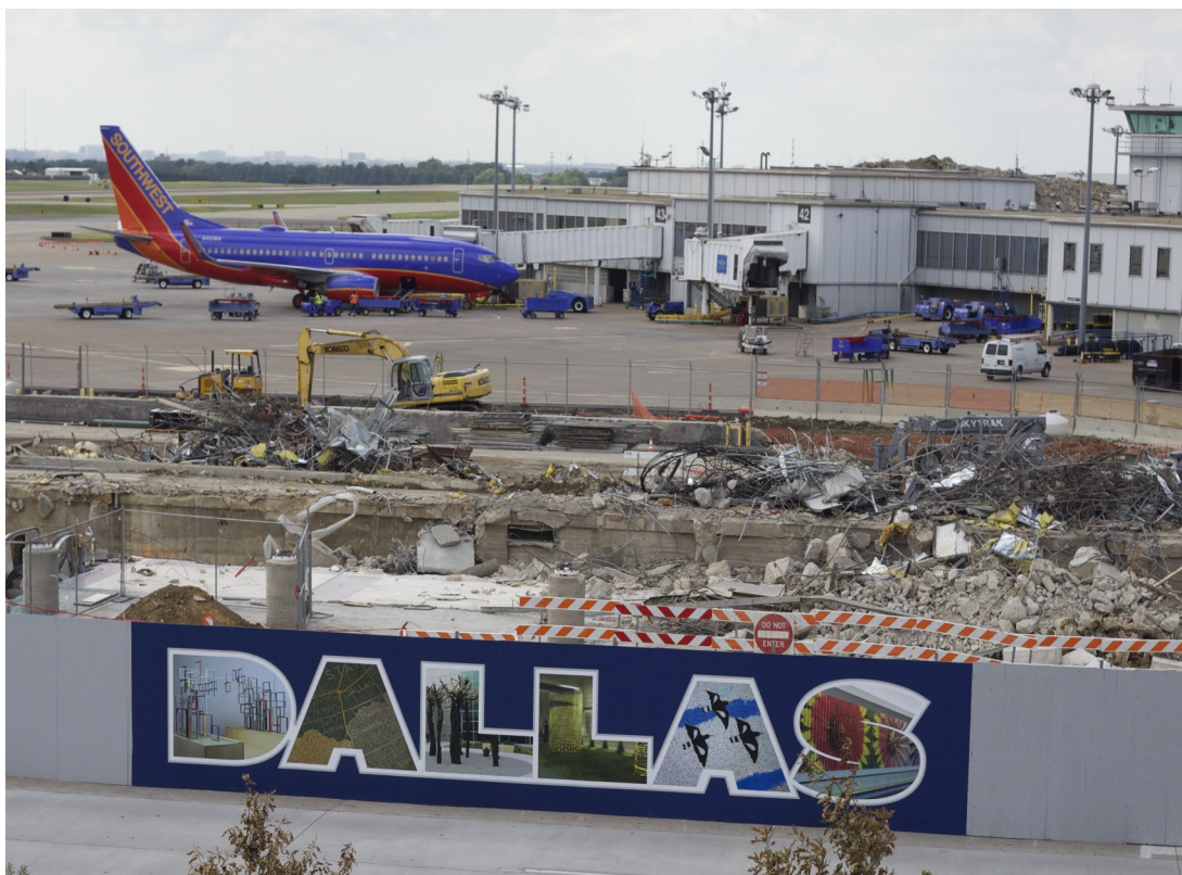
Photo above shows the demolition of the old baggage claim hall.
